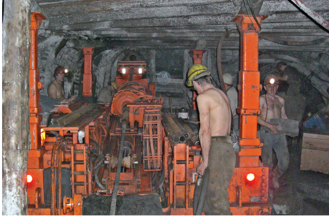
Figure 2: Directional drilling of horizontal gob boreholes underground at the Belozorskaya Mine in Ukraine.
